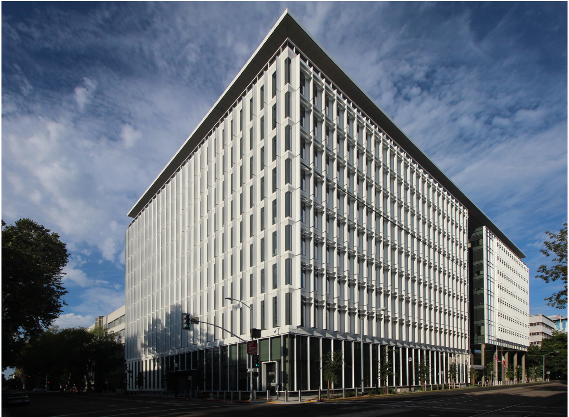
Photo Credit: Willis Construction Co. Inc., O Street
