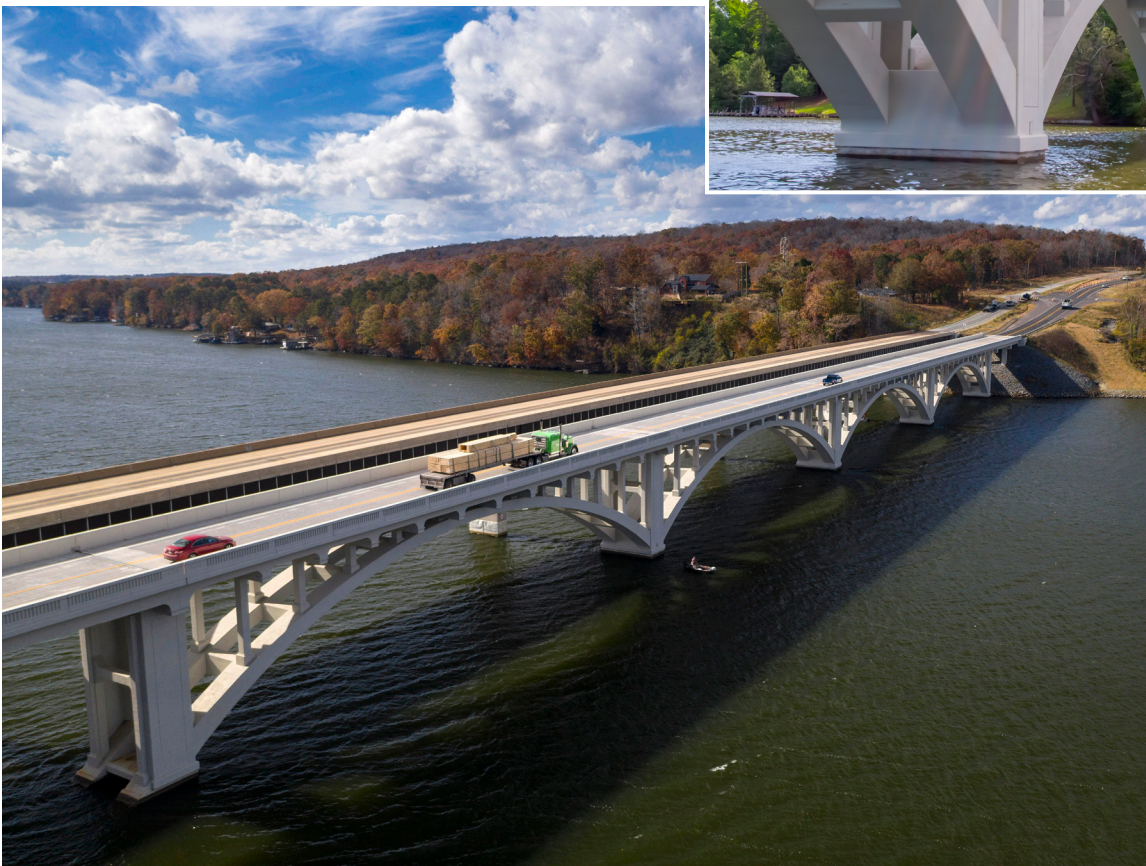
Photo Credit: AECOM., Swift Island Historic Arch Bridge Rehabilitation and Widening
