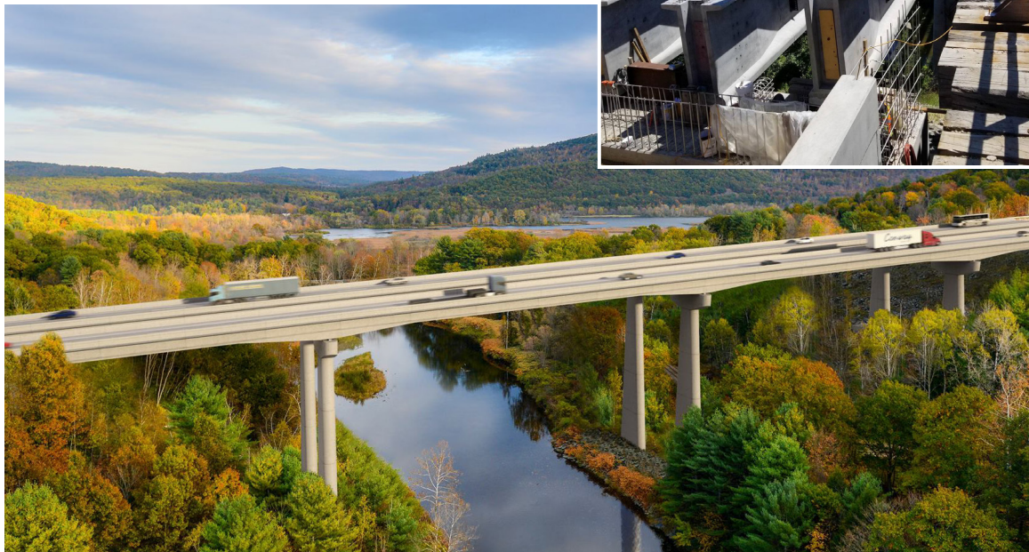
Photo Credit: JP Carrara & Sons, Inc., Rockingham I-91 Bridges 24N and 24S - IM 091-1(66)
