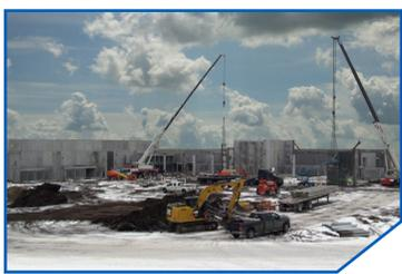
Wells Concrete provided 1,550 precast members including columns, beams, and architectural and structural wall panels boasting sandblast and waterwash finishes. 1,800 members of hollowcore were provided by Gage Brothers and then erected by Wells Concrete.
