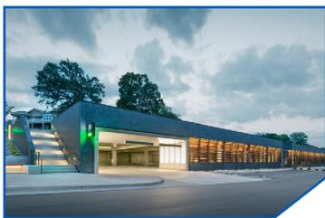
The Mill Street Parking Ramp included construction of a new 385-stall, 93,700 SF parking structure for the downtown City of Wayzata. Work consisted of a cast-in-place concrete with a post-tensioned cable 2nd floor deck. Exterior façade consisted of precast panels with a thin-brick facing, factory finished metal wall panels and decorative ipe wood cladding.
